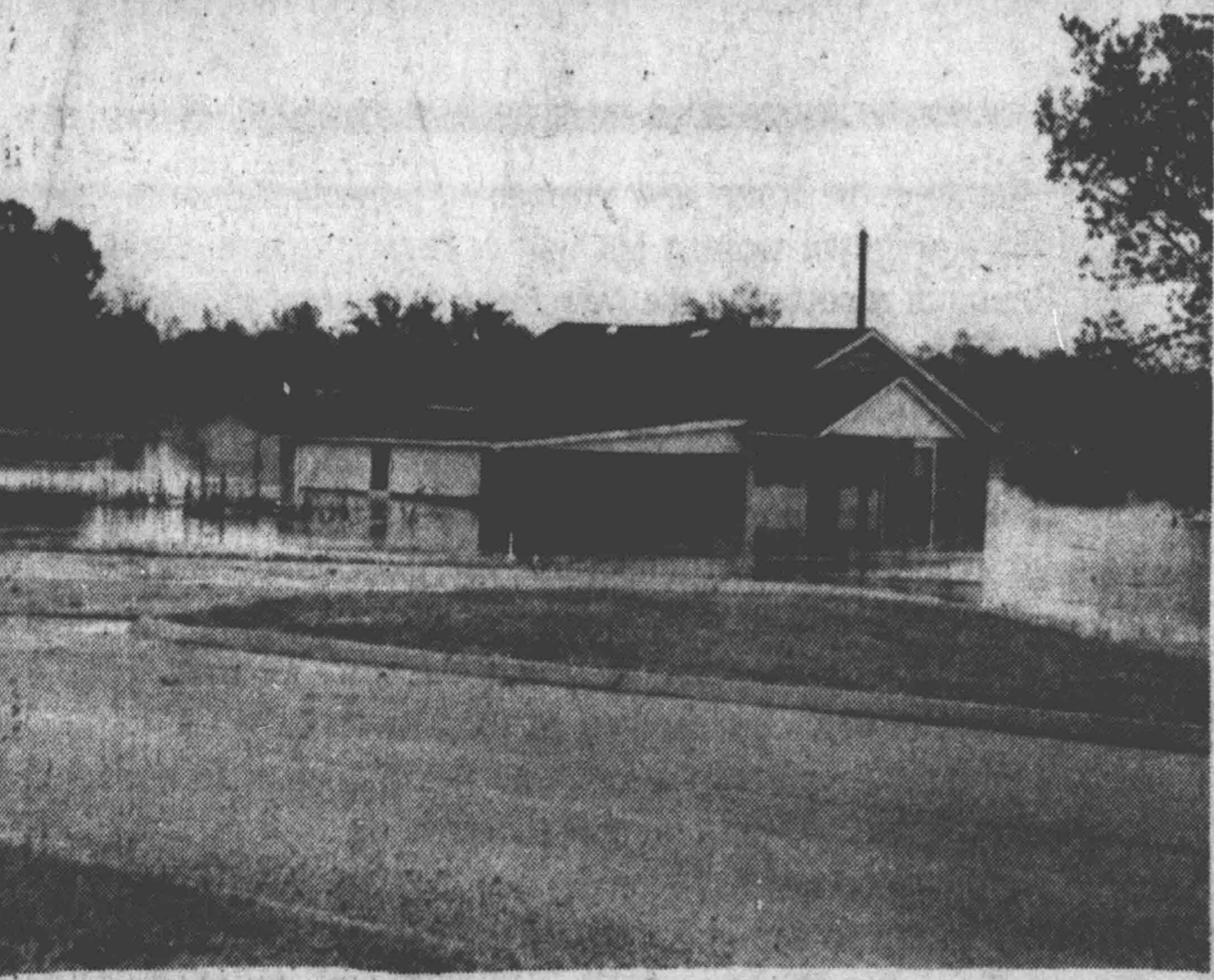
HALLS AREA FLOODING early Thursday of last week resulted from about six inches of rain in a few hours.
